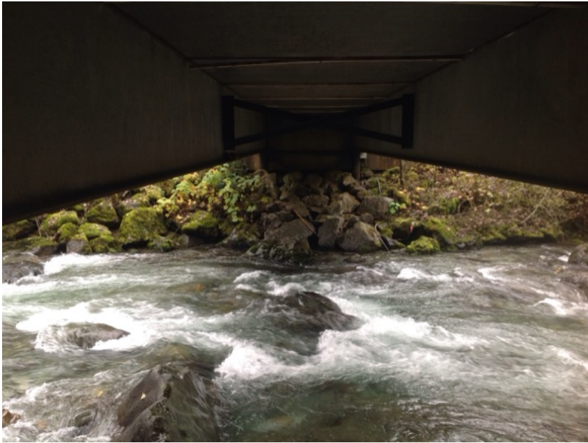
Left Bank Abutment when facing downstream
