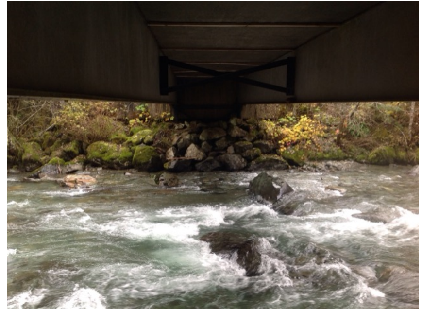
Right Bank Abutment when facing downstream
